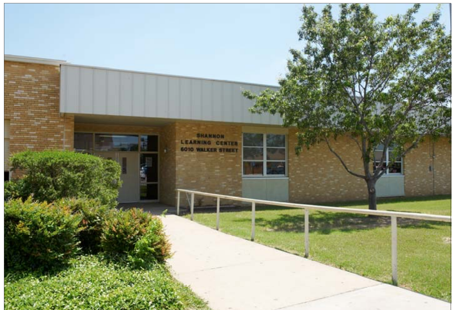
Daikin's VRV Heat Recovery system which allows simultaneous heating and cooling was chosen to replace decades-old HVAC system in the Shannon Learning Center.
